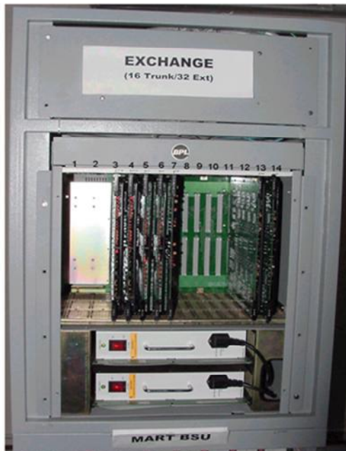
SLOT 3 & 4 : CPC CARDS SLOT 7 : DTR CARD SLOT 5 & 6 : ALC CARDS SLOT 13 & 14 : E&M CARDS
